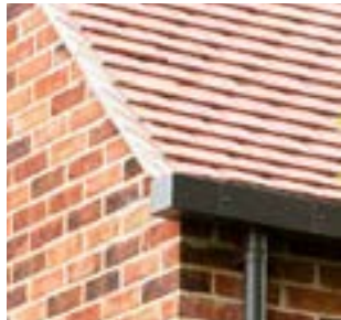
Mortared roof verge
