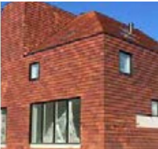
Tiles across roof and walls
