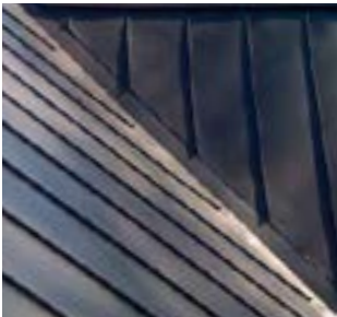
Folded standing seam roof and walls
